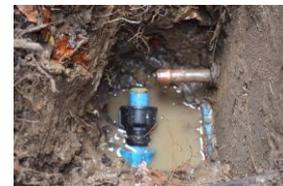
More gas was used to pinpoint the area of the leak. We dug down about a metre to find the poly pipe. The water was re-engaged to assist in the exact location of the leak.
